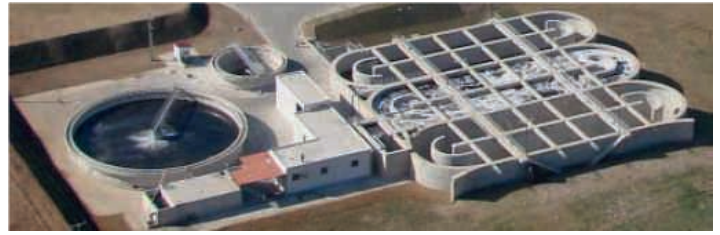
Complete Biological Treatment Plant
